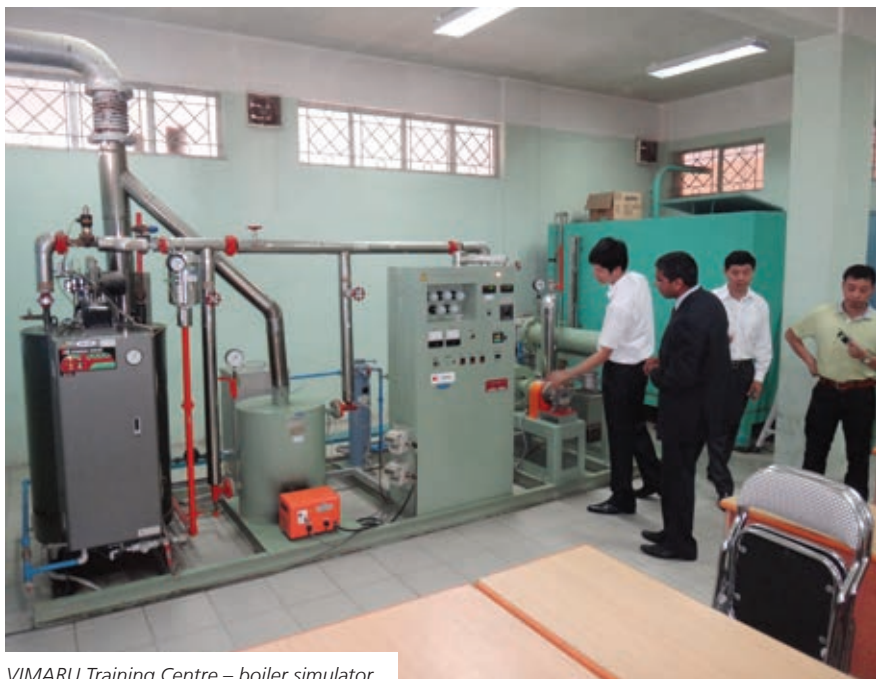
VIMARU Training Centre – boiler simulator.
