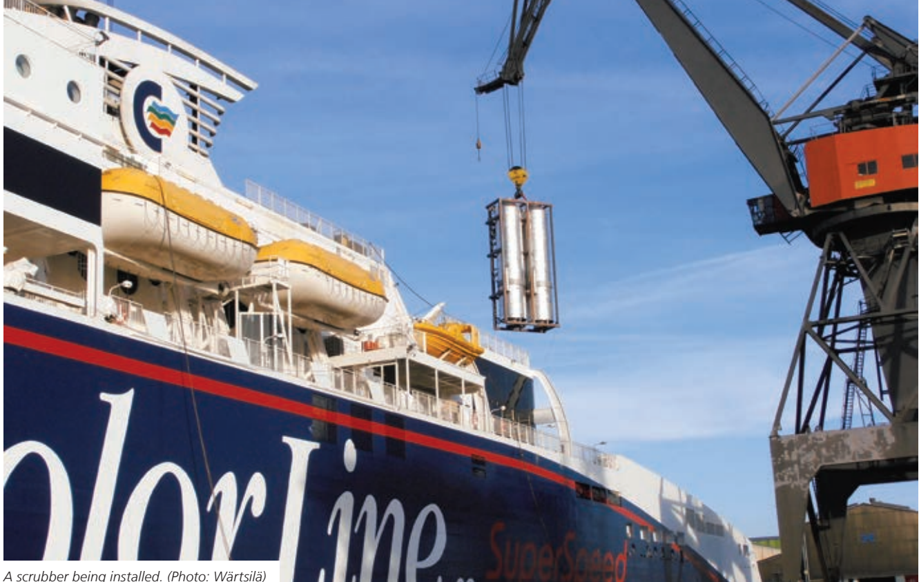
A scrubber being installed. (Photo: Wärtsilä)
